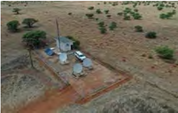
Aerial view of the CRF, showing the CGS, IDC GCI and AFTAC VSAT satellite antennas, AFTAC solar panels, the CRF building in Boshoff.
